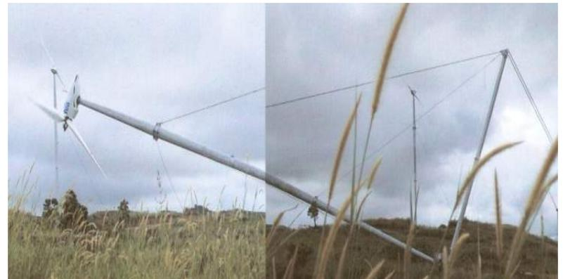
bine. The winching arrangement also allows the turbine to be raised to the vertical without the need for an external crane, which is a considerable advantage in remote areas.
